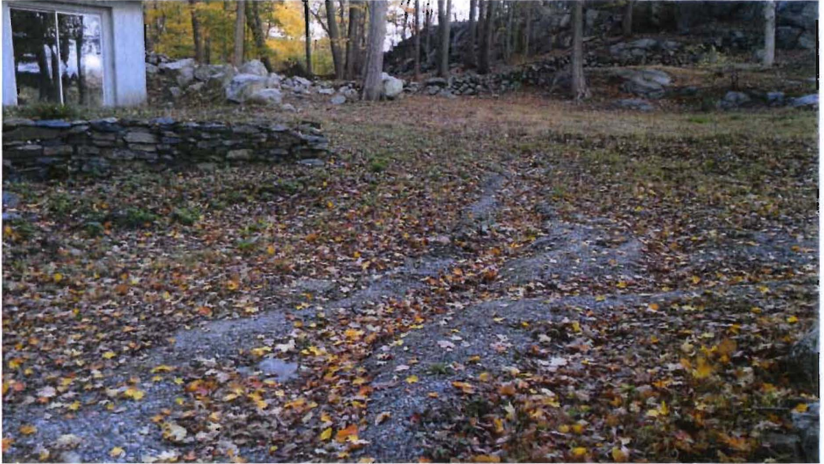
Eroded rills in existing driveway
