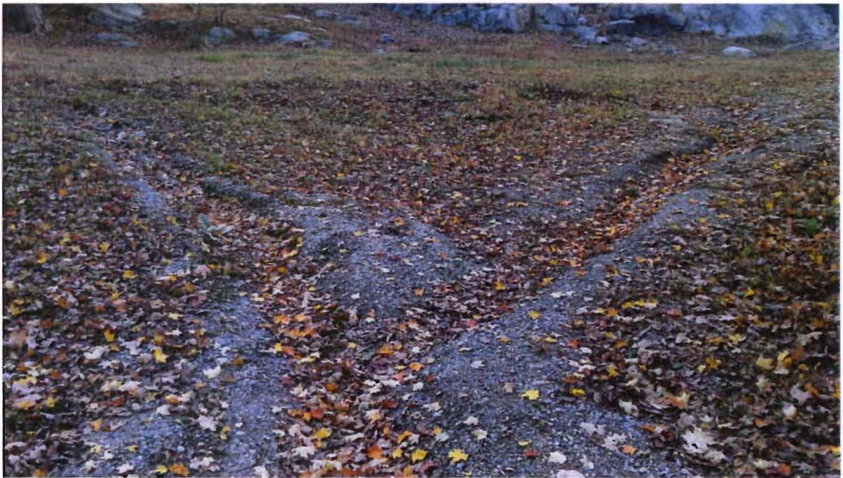
Eroded rills in existing driveway
